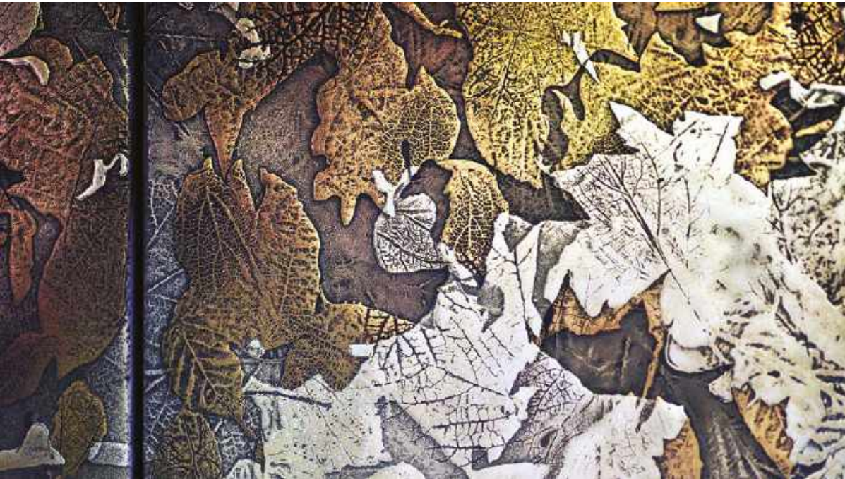
Left: The bronze clad detailing on the lift doors are cast from moulds of leaves found within St. James' Park.
