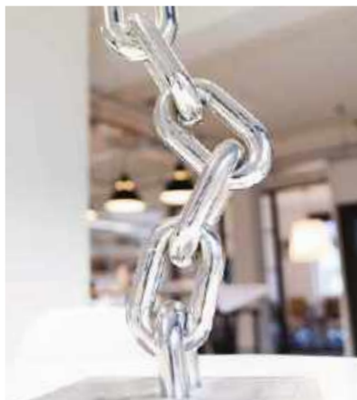
The huge chain down-pipe appears to anchor the building into the city, it also functions as a guttering system from the canopy to the flower bed below.
